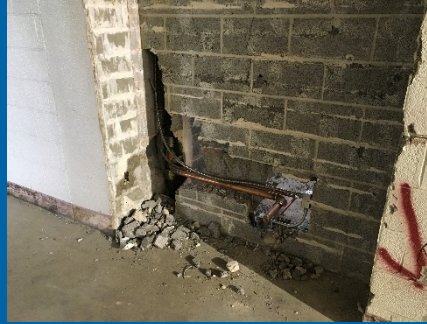
In Wall Plumbing and Electrical Rough for New Water Fountains
