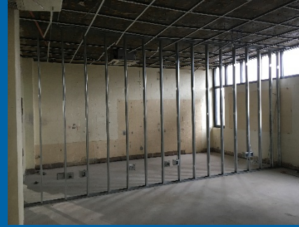
New Framing and Electrical Wall Rough In
